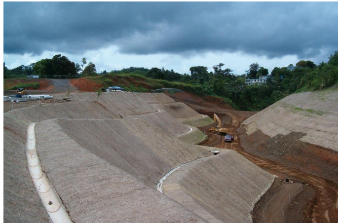
2. Chiclana Creek Restoration - San Juan, PR 2005
