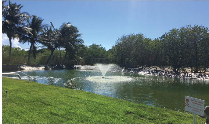
1. Retention Lagoon Wastewater Guánica, PR 2019
